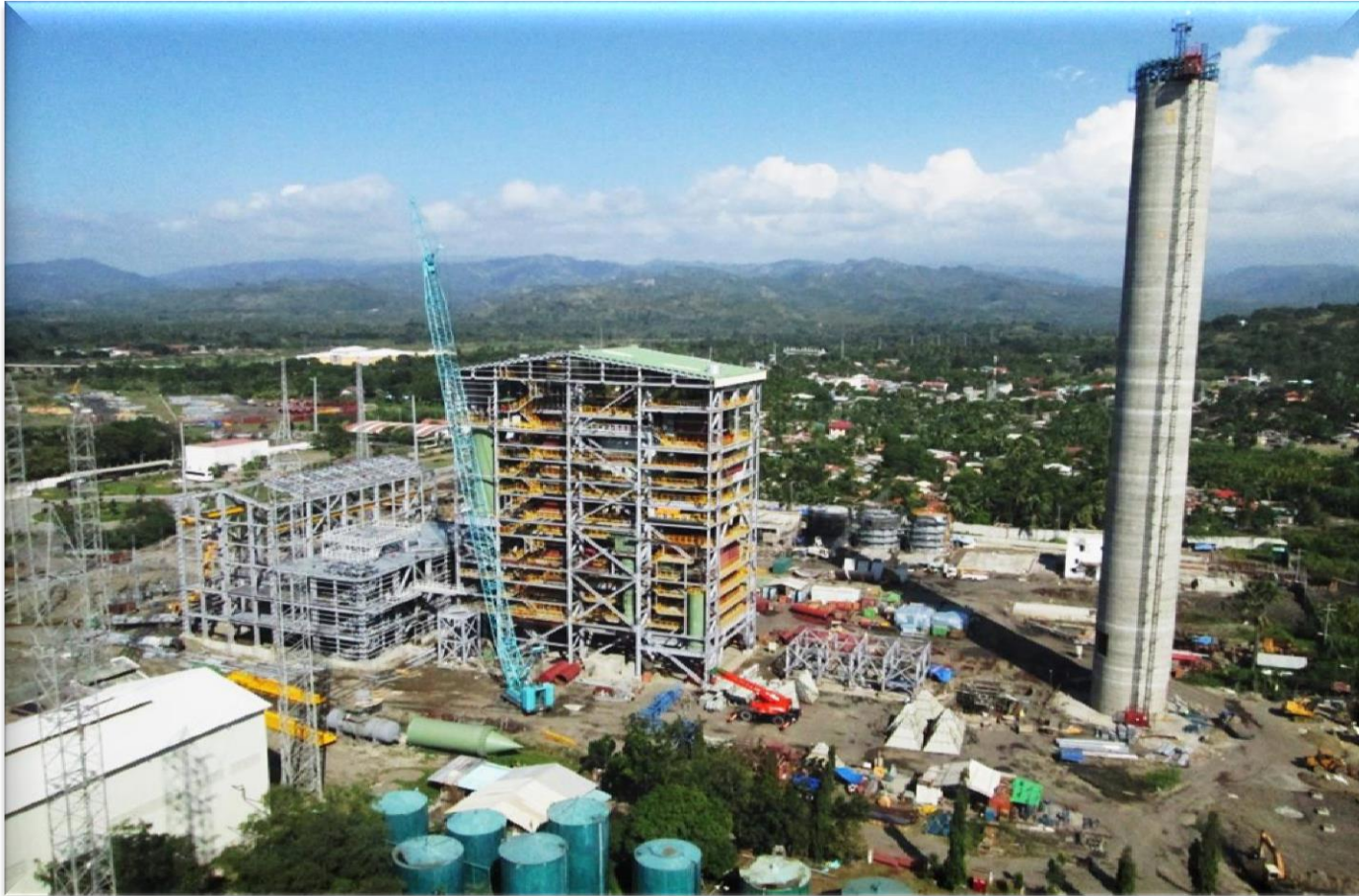
Toledo Power Company (TPC) 82-megawatt Expansion Toledo City, Cebu
