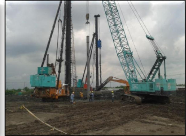
Piling at Boiler Area using Machine #2
