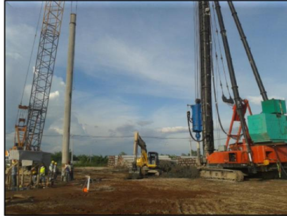
Piling at Boiler Area using Machine #1
