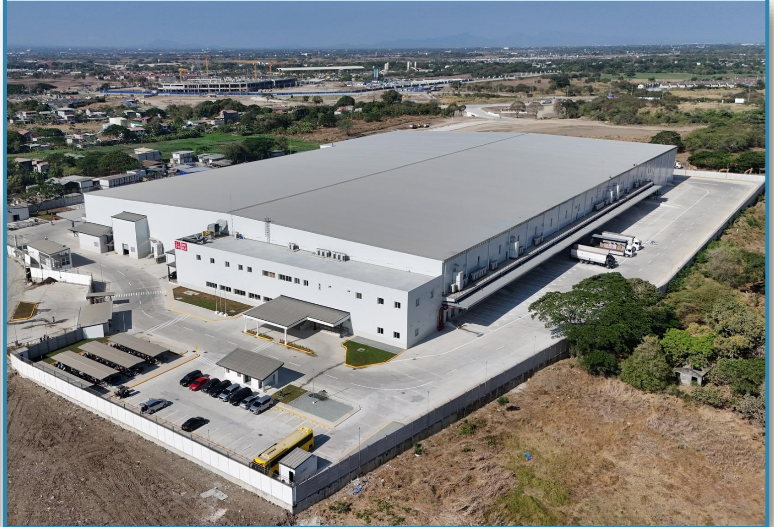
Uniqlo Logistics Facility in Riverpark, General Trias
