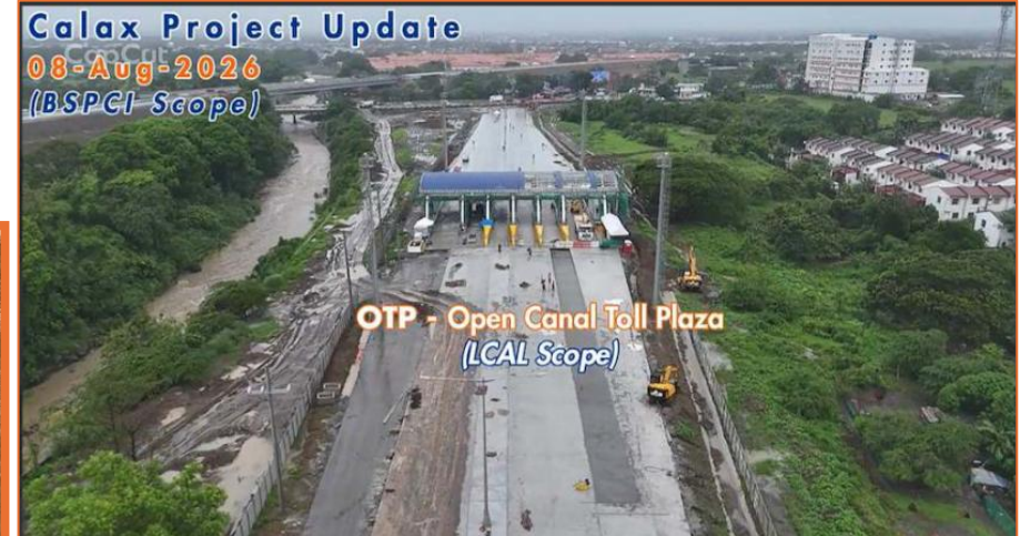
Open Canal Toll Plaza
