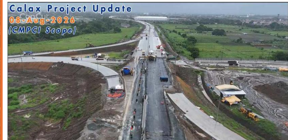
Open Interchange Bridge
