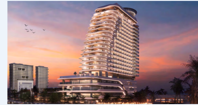
Landco's The Spinnaker earned international recognition as the Best International Sustainable Residential Development
