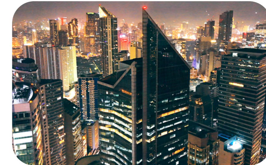
GT Tower along Ayala Avenue, Makati City
