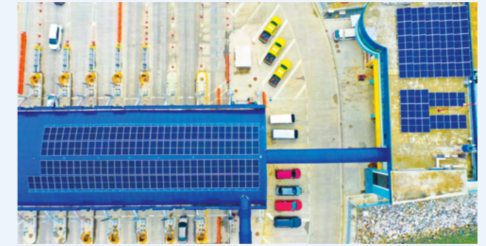
Solar panels at toll plaza
