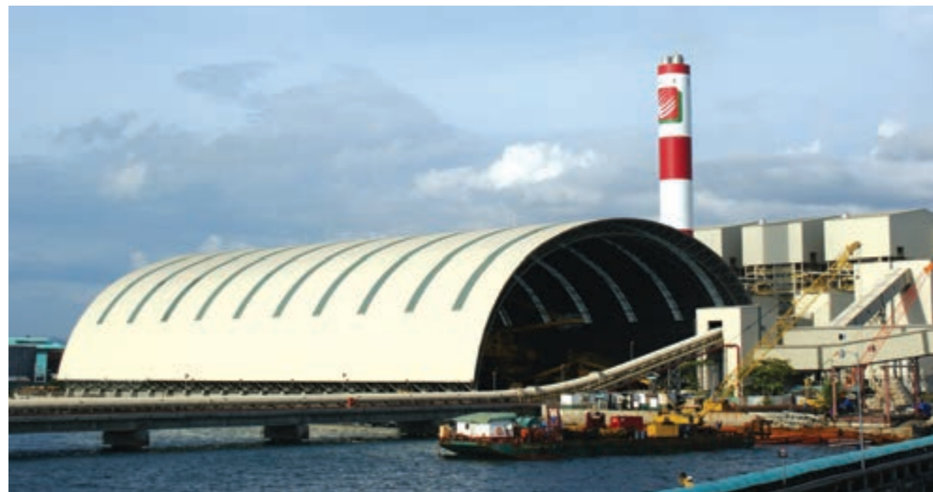
246-Megawatt Cebu Energy Development Corporation (CEDC) Power Plant in Toledo, Cebu
